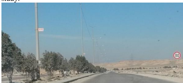
Figure 13 Labels fixed on electrical columns along Ring Road in Al-Najaf city.
