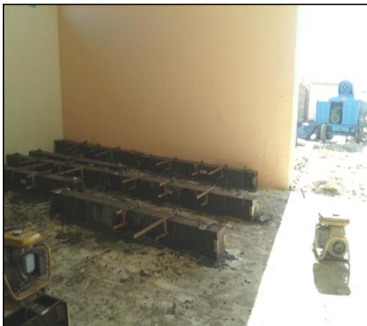
Figure (4). Concrete Casting for specimens
