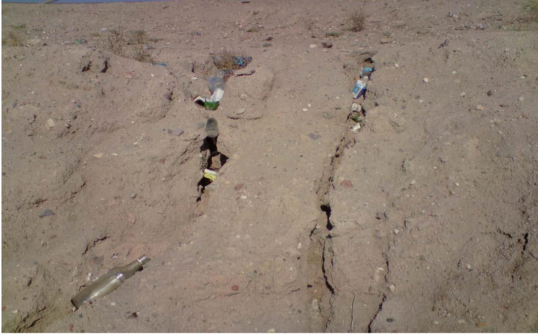
Fig.(2) Study embankment with remarked gully erosion
