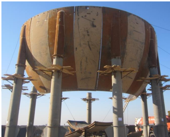
Fig.(1): Spherical LPG steel tank in Maysan during construction
