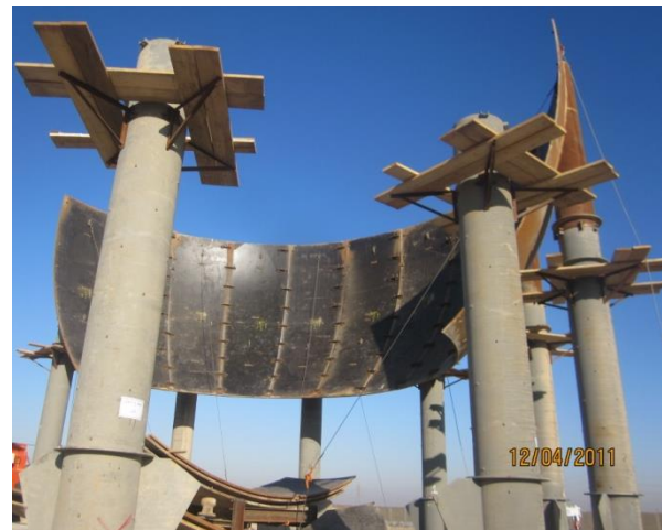
Fig.(1): Spherical LPG steel tank in Maysan during construction
