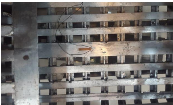
Fig (4) Installing sensor in the middle of ship hull.
