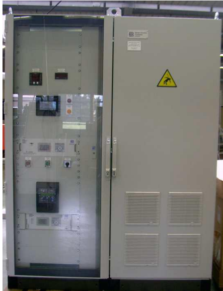
Fig.2 Excitation system panel
