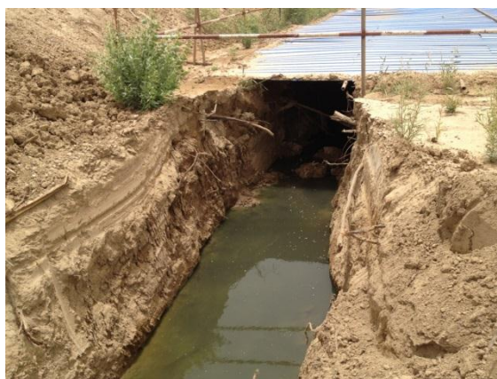
Figure (2) Chinese camp -underground septic tanks with directly wastewater discharge to the river.
