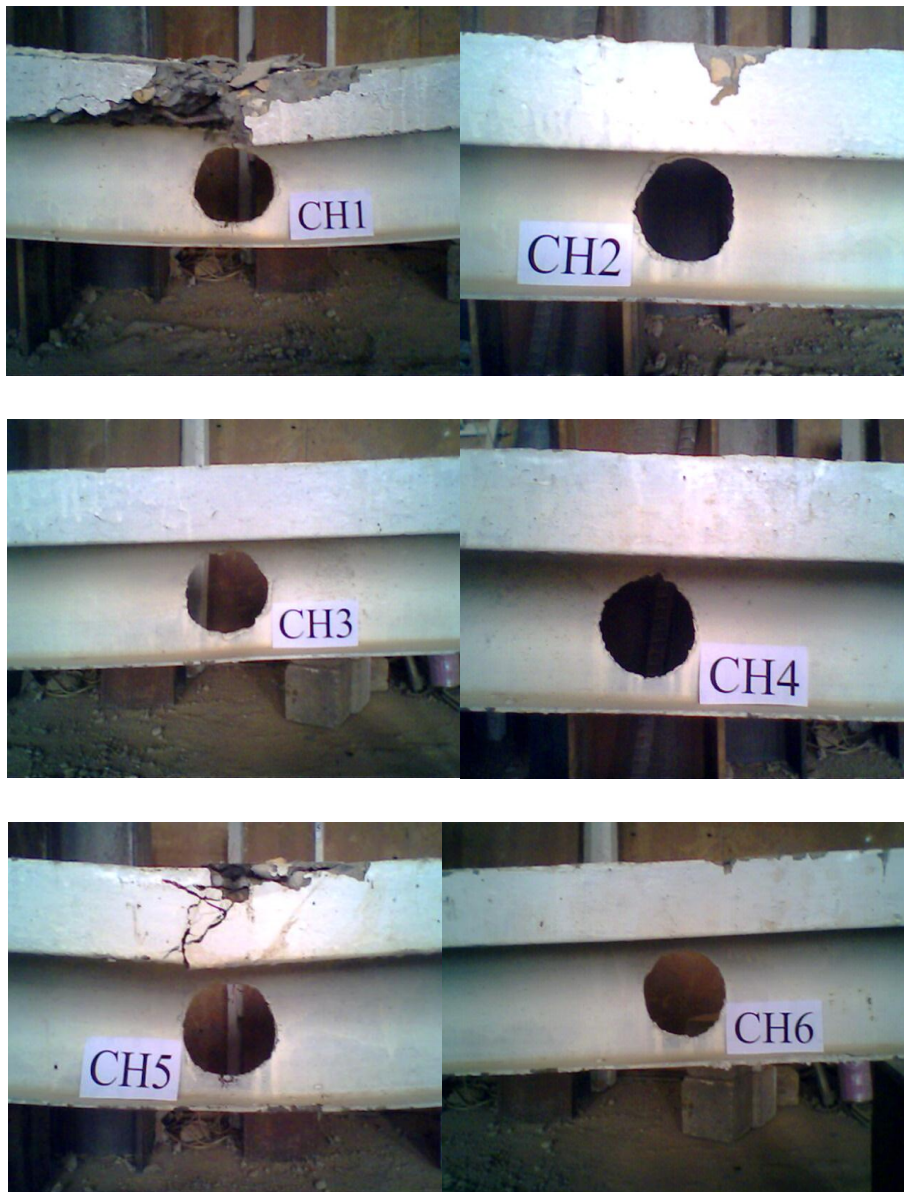
Figure (5): Openings at failure
