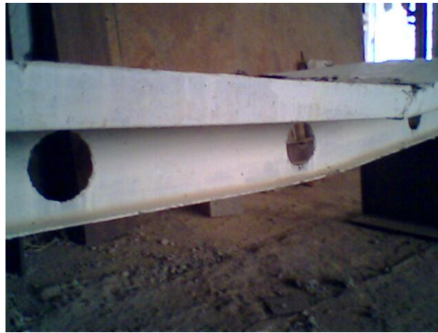
Figure (7): Typical failure mode ( Beam CB3)
