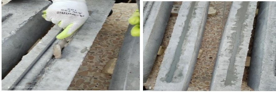
Figure 7: Strengthened beams using NSM with geopolymer
