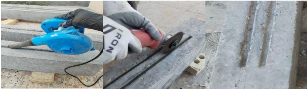
Figure 5: Preparation grooves stages
