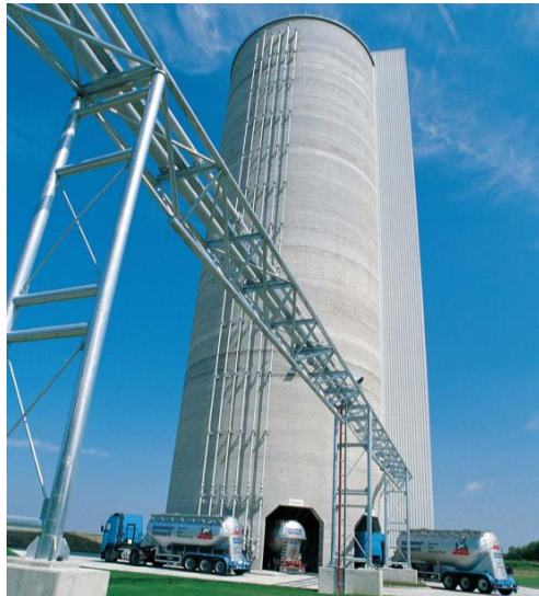
(a) Circular Silo
